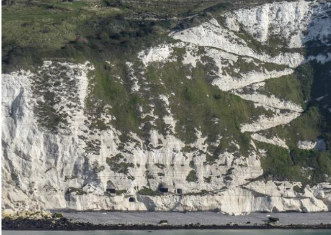
The Langdon Stairs zig-zag down the right-hand side of this picture taken from a ferry in September 2018; the searchlight positions, ladder to the beach and rockfall can be seen in the lower middle of the picture
