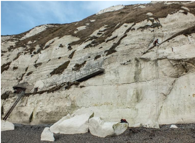
A closer view of the last zig-zag in December 2016; one of the remaining searchlight positions and the final metal ladder to the beach can be seen to the left of the picture and the rockfall debris and the resulting gap in the final zig-zag can be seen on the right of the picture
